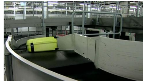
Figure 1 Transportation by belt conveyor
