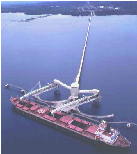
Figure 2. Example of a Jetty Conveyor Feeding the Ship Loading Equipment. The length of the conveyor is 2 km. and the transport capacity is 4200 MTPH. (Kaltim Prima Coal Mine).
